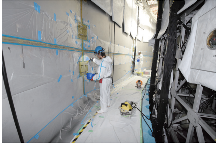
Figure 5: Sealant work on the SK tank wall being conducted from the floating floor. An outer detector PMT can be seen at the right side.
